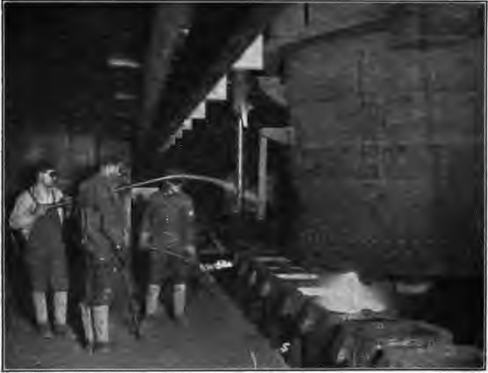
FIG. 116.—Pouring the molten steel into the ingot molds.
